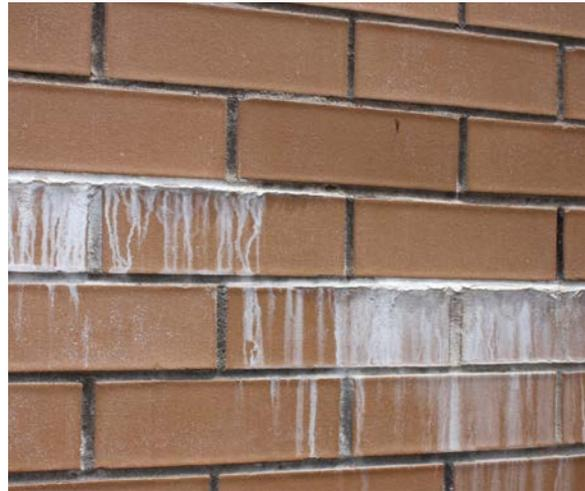
using Efflock in mortar that is compiled with washed sand (without clay) and hydrated lime as a plasticiser. It was found that the accelerant effect can be avoided by substituting lime with clay, but the use of clay should be signed off by a structural engineer and/or tested under the relevant standard (i.e. AS 3700) to confirm satisfactory performance.
