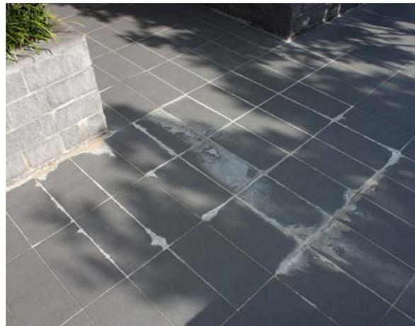
Timber frame and cement sheet structures should be constructed to fall. Tile screed should be reinforced and un-bonded with a separation layer. Tile screed may be able to be omitted altogether by expressing sheet joints throughout the tiles with caulked expansion joints or by bridging lateral movement cracks with a decoupling system (subject to manufacturers' recommendations).
